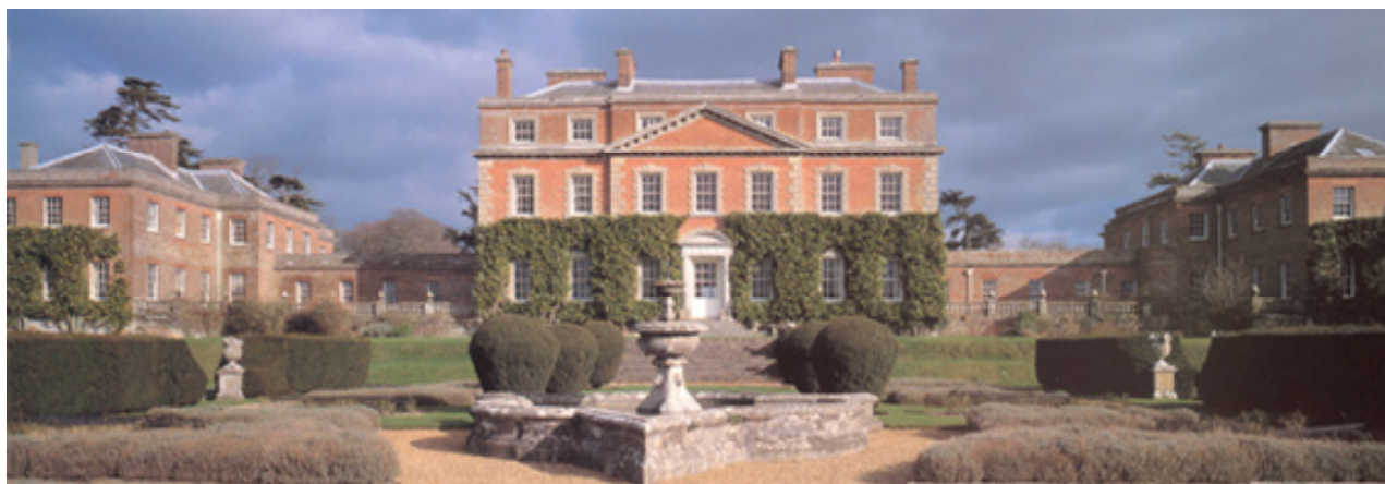
A view of the west front of Trafalgar Park
